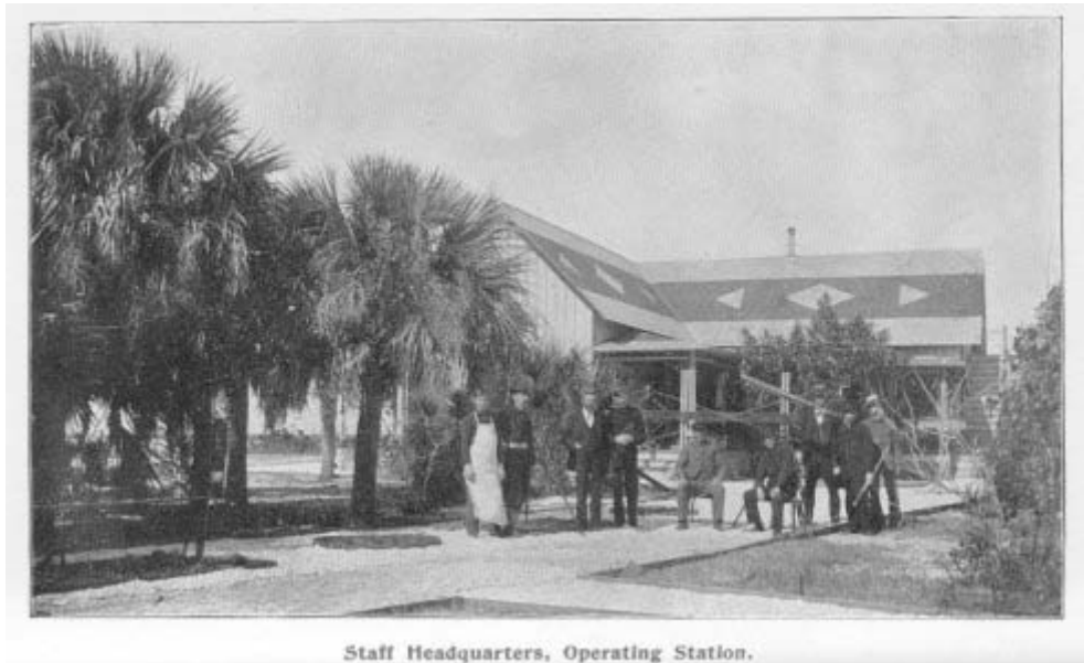
Staff Headquarters, Operating Station
