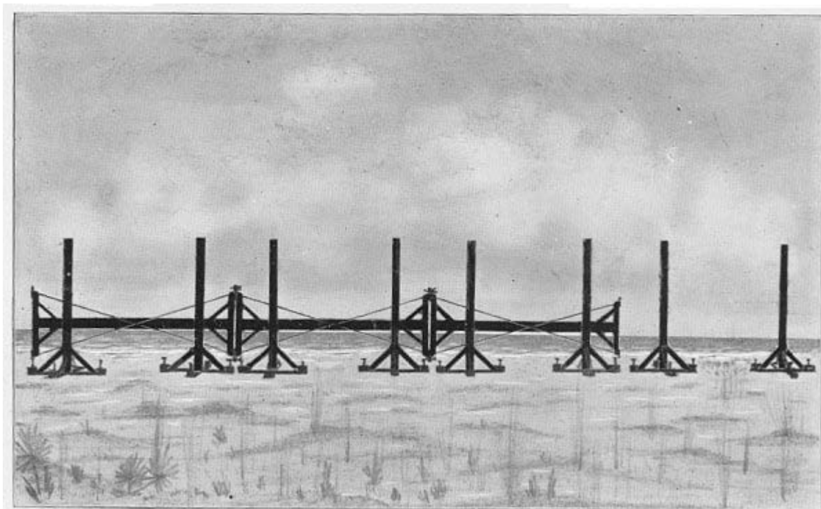
Away Down on the Standards.
