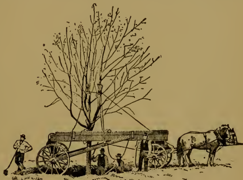
149. The tree ready to lift.
