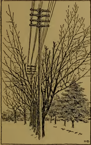
164. Trees ruined to allow of the passage of wires.
