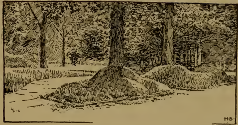
173. A method of saving valuable trees along streets on which heavy lowering of grade has been made.
